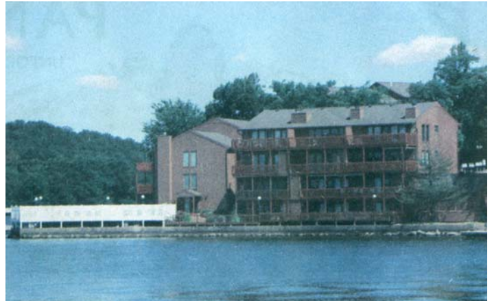
This is one of the two Lake Valley Condominium buildings constructed below the 670 contour line, which Ameren UE claims does not comply with their regulations. Nancy Hogland photo.
